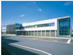
Internal broaches factory
