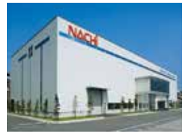
Special steel melting factory
