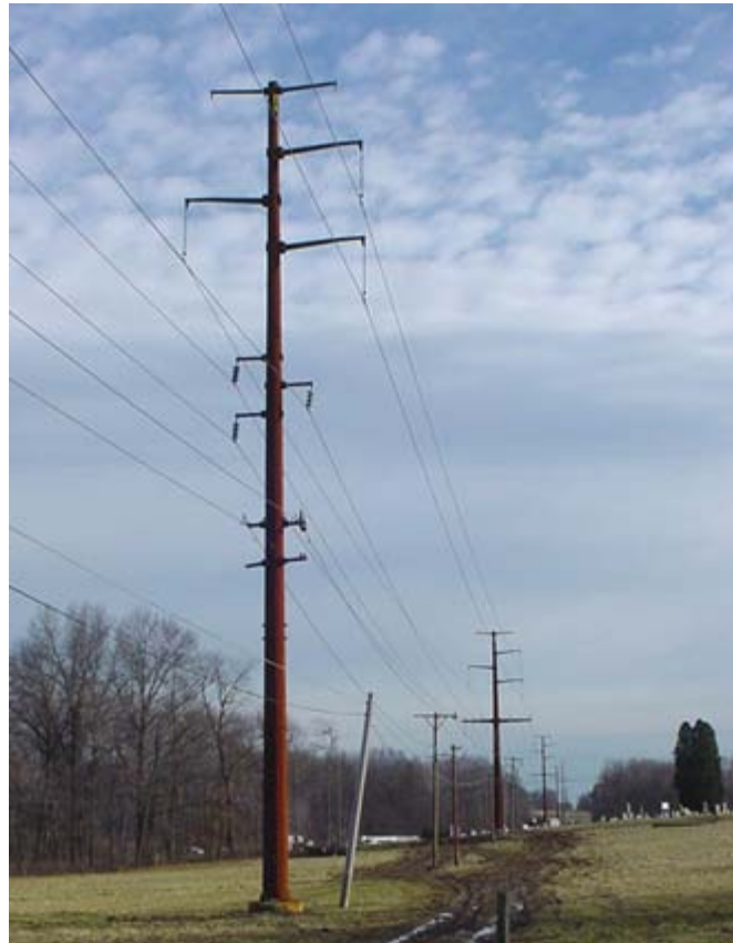
Single circuit delta arrangement with distribution underbuilt (suspension)
