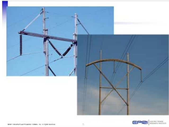
Single circuit, wood H-Frame design with standard and curved cross arms. (suspension)
