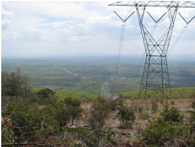
Single circuit steel tower (suspension)
