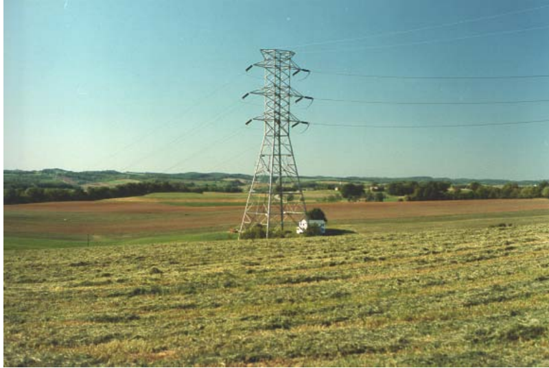
Double circuit steel tower (strain)
