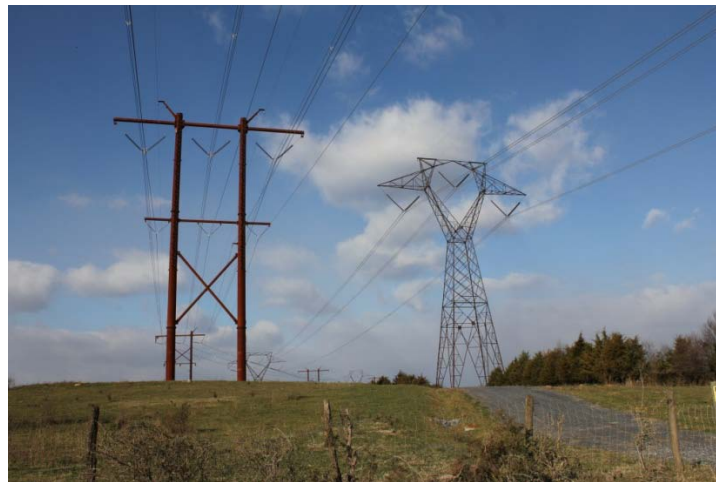
Single circuit, steel H-Frame design with underbuilt alongside a single circuit steel tower (suspension)
