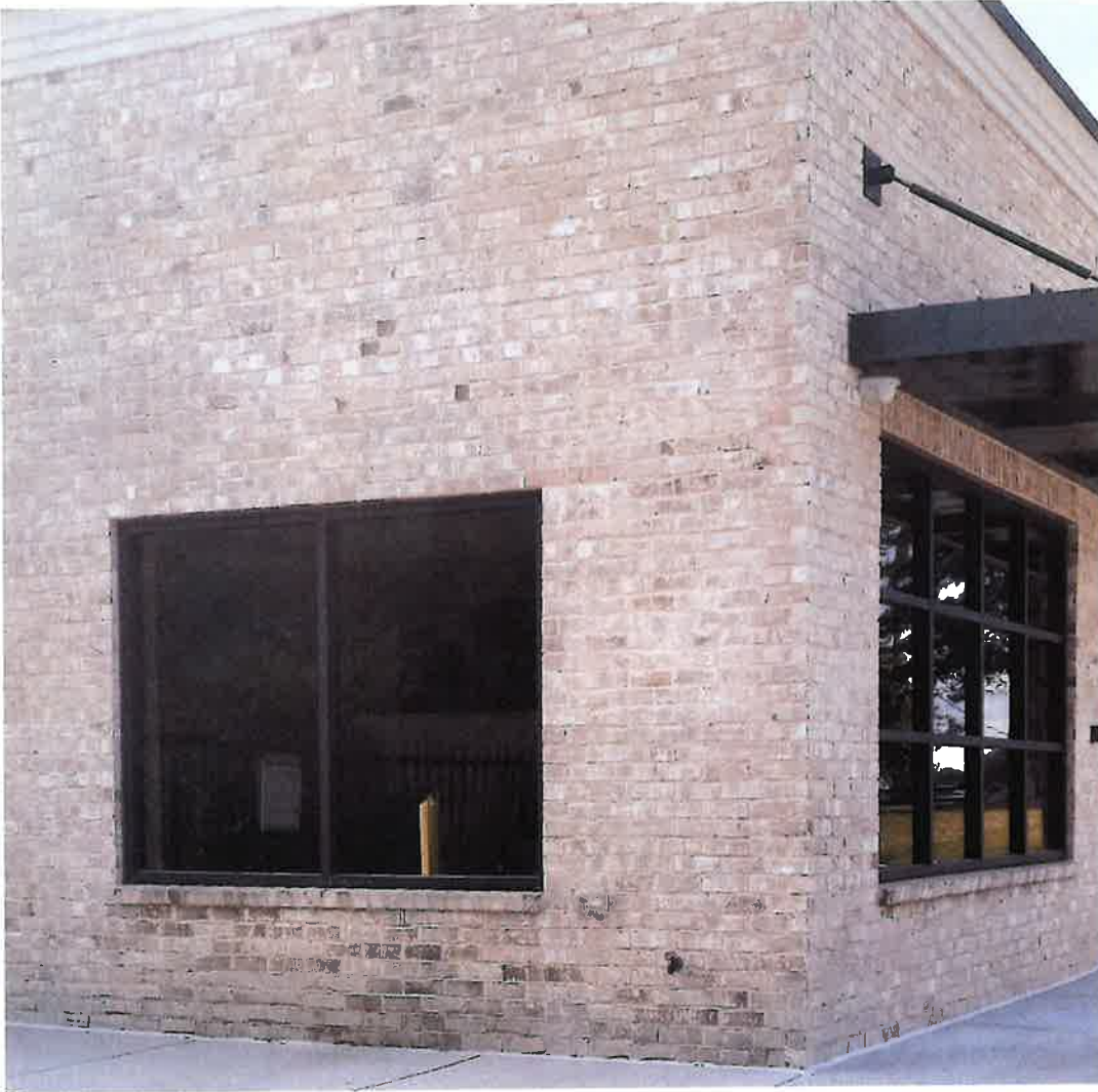
Exterior Brick material facing road frontage
