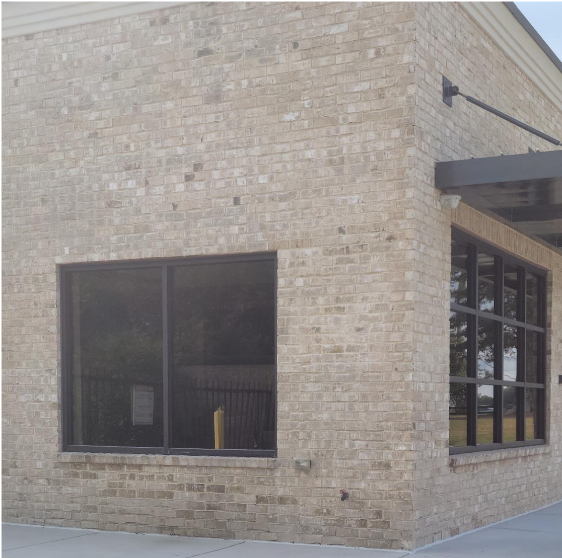
Exterior Brick material facing road frontage
