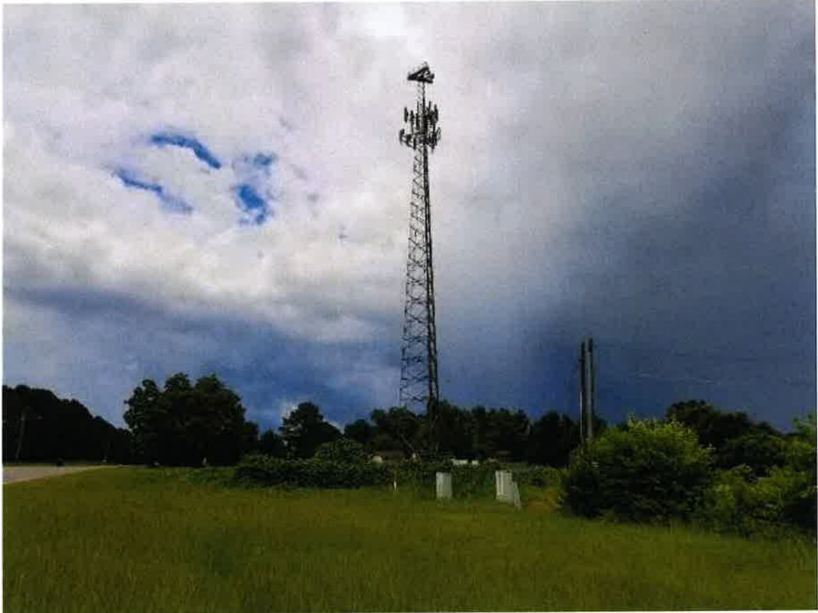
View of Telecommunication Tower From Highway 41 and Highway 41 Loop
