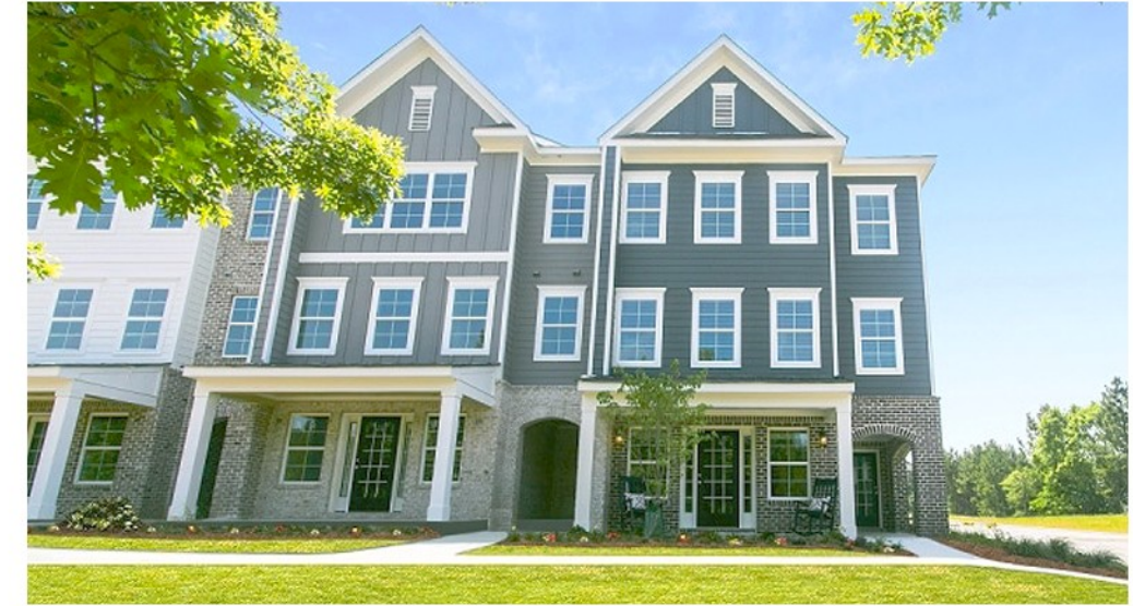
FRONT DOORS TO LOWER UNIT AND UPPER UNIT
