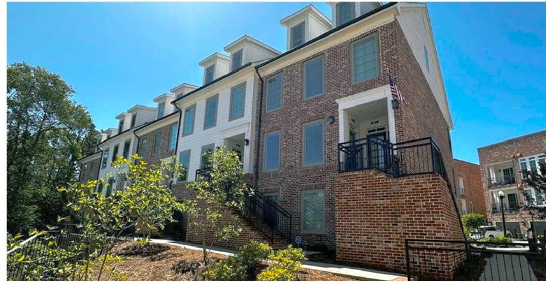
FRONT ENTRY AT LEVEL TWO
