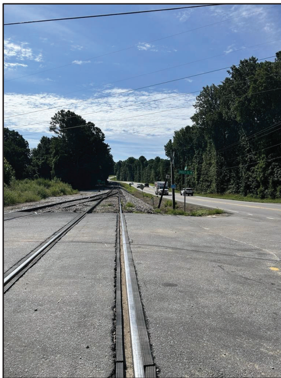
SR 60 South Approach
