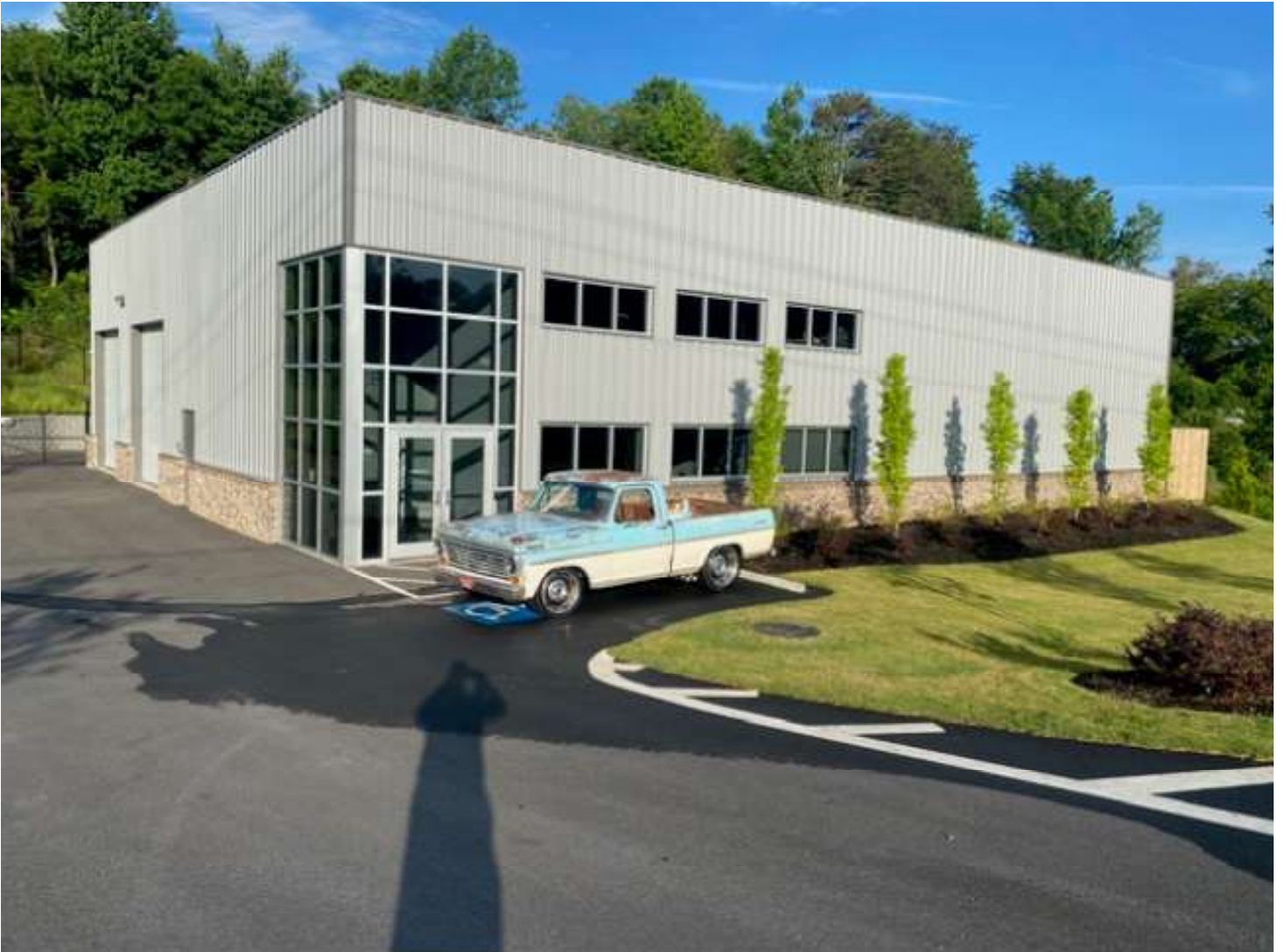
Photo of Existing Building
