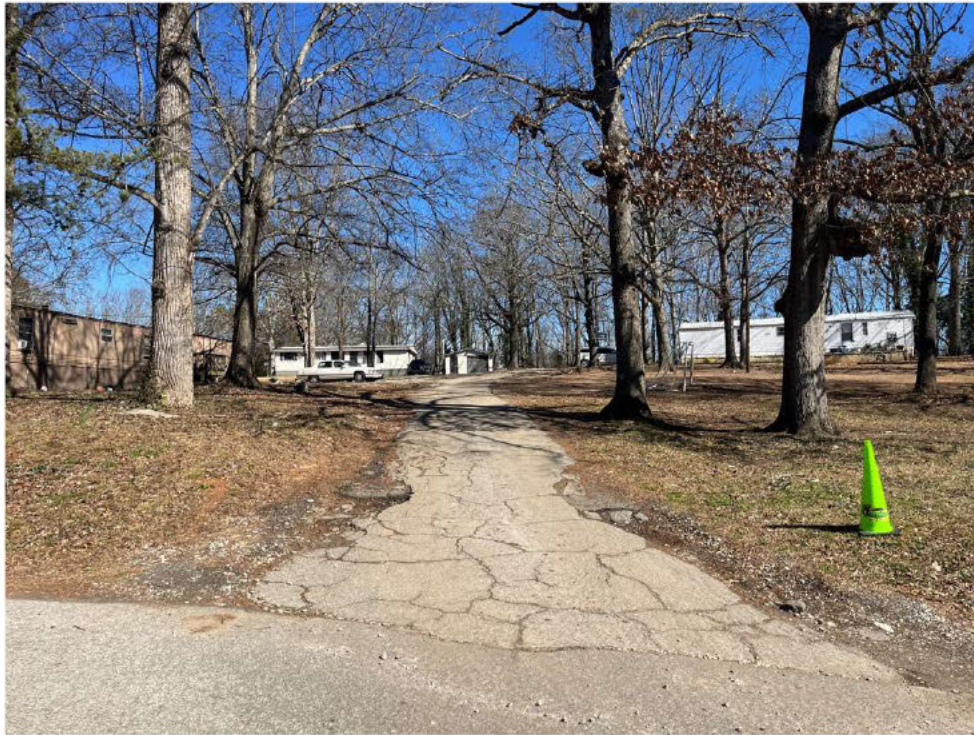
Site Photograph 13 – Looking north along the easement from the terminus
