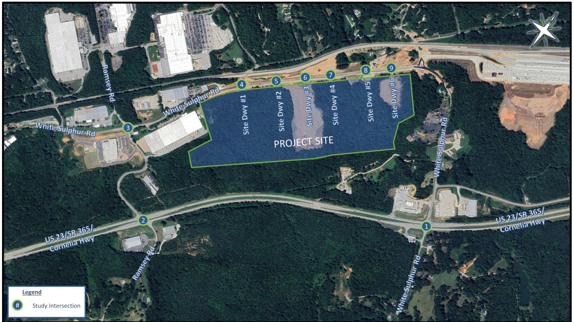
Figure 1.1 – Aerial View of Study Area
