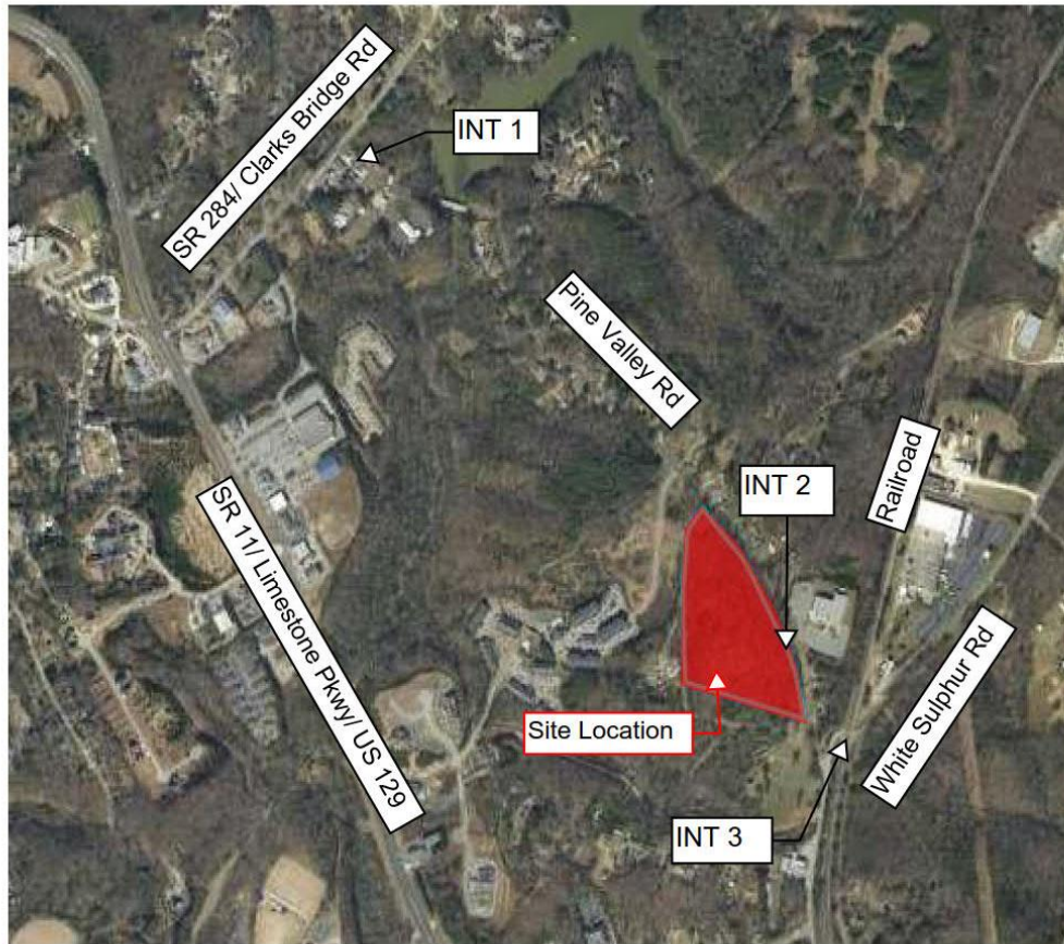
Figure 2 Aerial of Study Area
