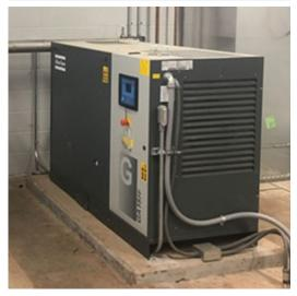
The compressor can be located indoors for weather protection and ease of maintenance in a climate-controlled environment
