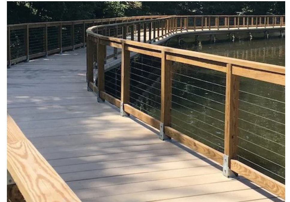
Wood cable railing along Logan Lake Boardwalk
