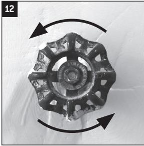
12. Once the water has stopped sputtering as the air has been bled from the line, shut off the previously opened faucet from step 2.
