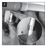
8. Connect the plug on the end of the long flat wire coming from Control Panel to either set of prongs on the Leak Sensor, pushing until plug snaps in place. Then place Leak Sensor on the floor at the base of the water heater — in the water heater pan if there is one. NOTE: Additional Leak Sensors can be connected in series for added
