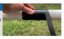
Pipe Repair Wrap can be a long-lasting solution, but it is not intended to be a permanent repair for pressurized applications.
