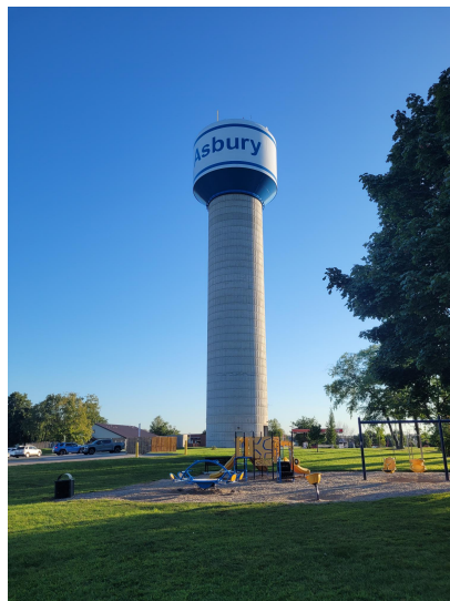
Figure 5.16: Standpipe water tower
