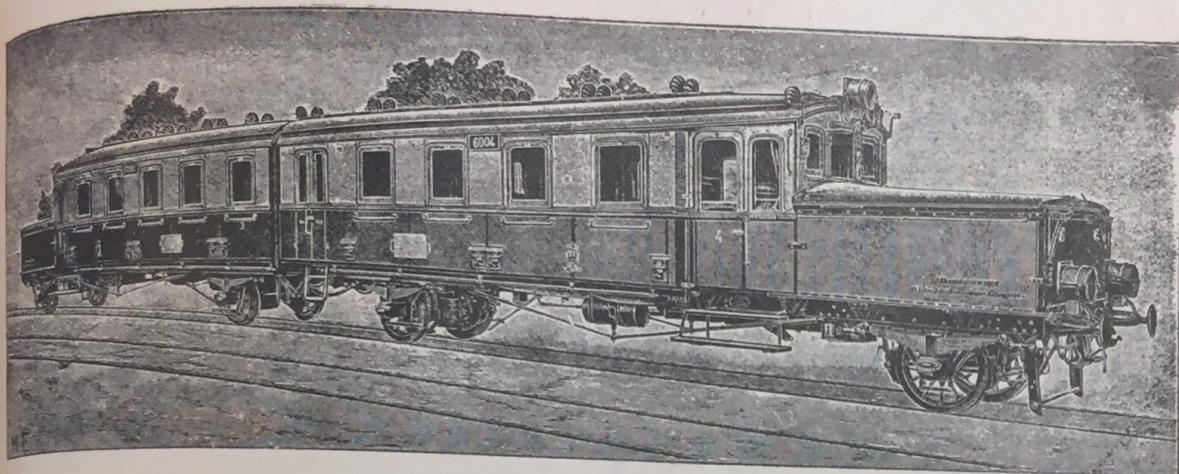
The Prussian Imperial Railroad now has in operation 19 trains of the type shown in accompanying illustration. These trains, composed of two cars, usually, have in front and in the rear a special tender carrying the storage batteries which are used for the propulsion of the odd looking "train." These trains
