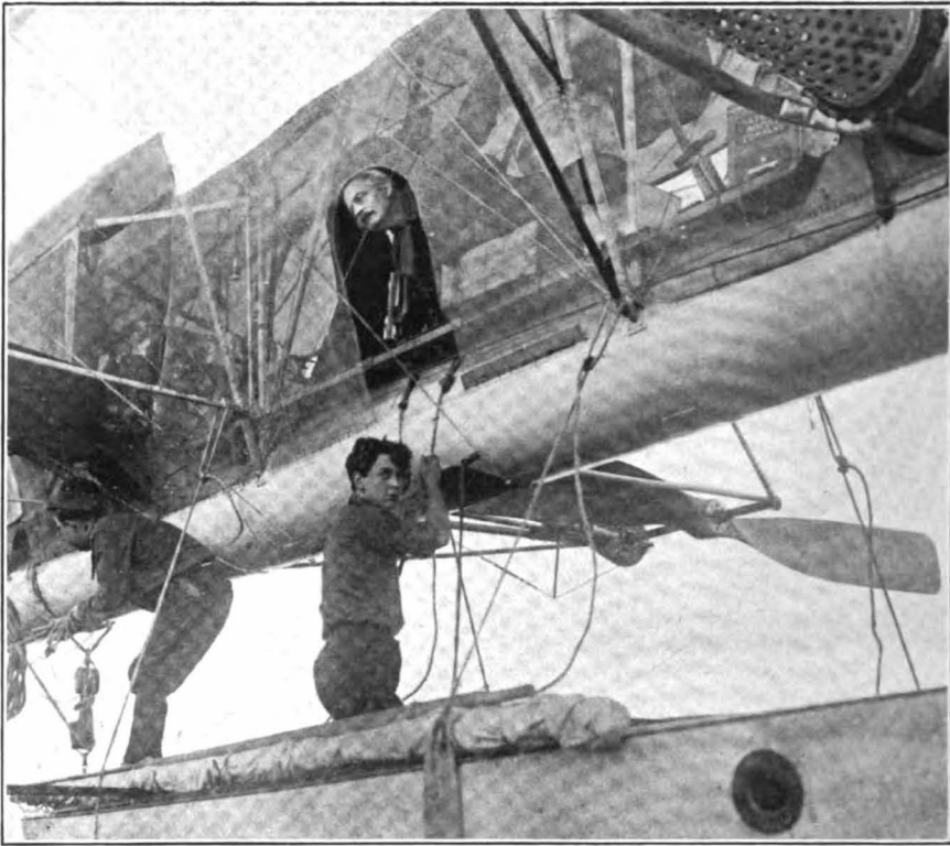
WALTER WELLMAN, IN THE AMERICA'S ENGINE-ROOM DOORWAY. LOUIS LOUD AND FRED B. AUBERT (ON RIGHT) ATTACHING THE LIFEBOAT JUST BEFORE THE DEPARTURE.
