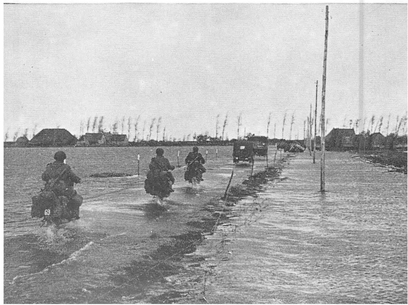
Troops drive forward over flooded roads towards Willemstadt. (British official photo)
