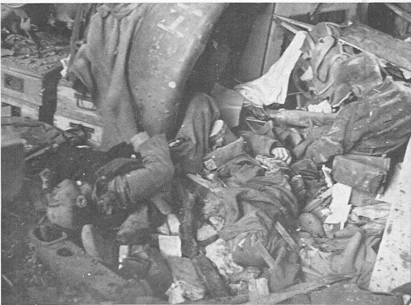
Inside view of a knocked-out German gun emplacement on Walcheren. ( British official photo )
