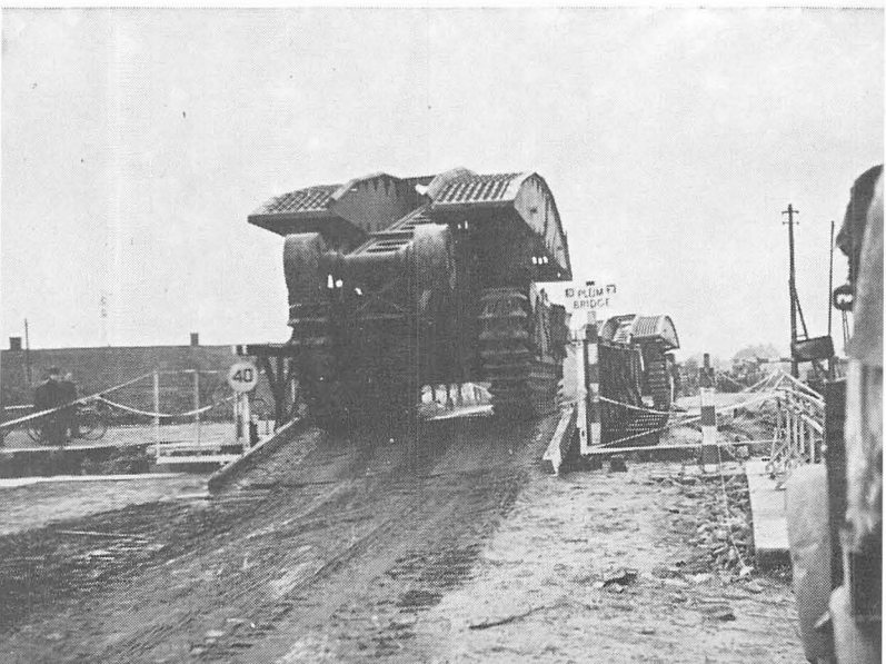
S. P. Bridges (Churchill bridge layers—"Jumbo") advancing over the canal. ( British official photo )
