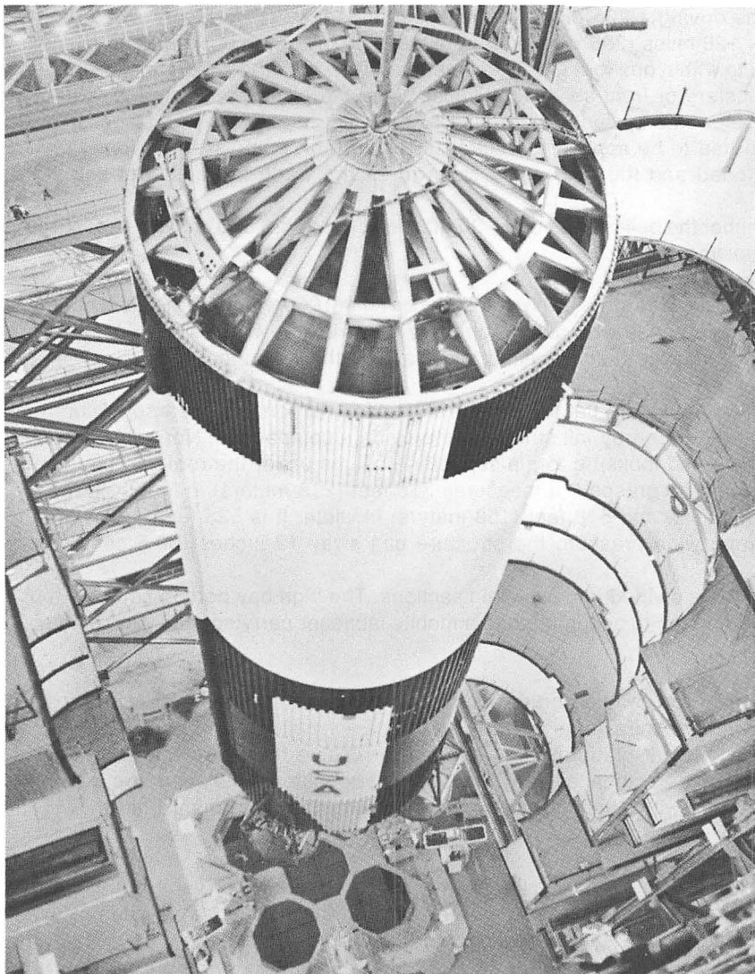
Precision control to the nth degree is required as this 250-ton (228-metric ton) capacity crane gently lowers the Saturn V first stage to the deck of the mobile launcher.
