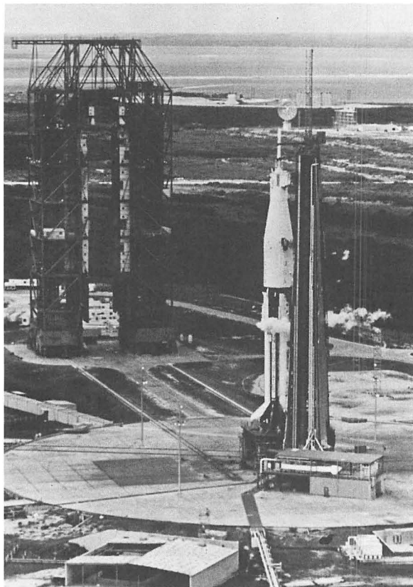
A Saturn IB booster stands at Complex 34, Cape Canaveral Air Force Station, poised to loft an Apollo command module into Earth orbit for performance tests.
