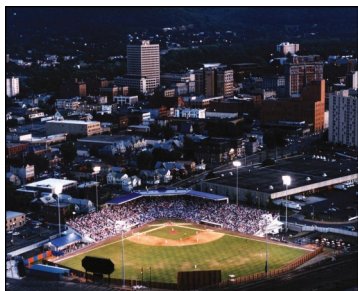
Binghamton Municipal Stadium seen from above in 1992
