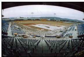
Municipal Stadium under construction in 1992
