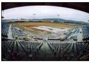
Municipal Stadium under construction in 1992
