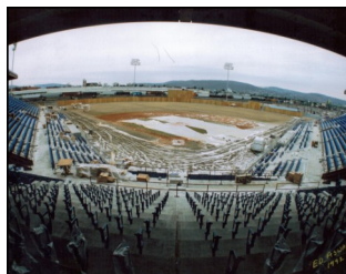
Municipal Stadium under construction in 1992
