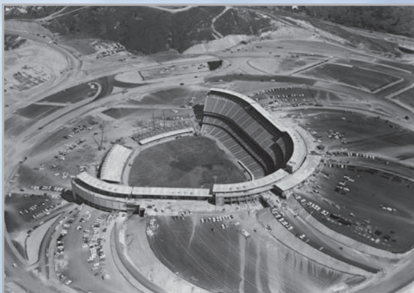
A birds-eye view of the Dodger Stadium construction and terraced parking at Chavez Ravine.
