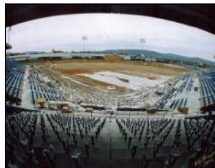
Municipal Stadium under construction in 1992
