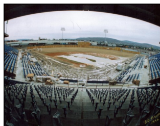
Municipal Stadium under construction in 1992
