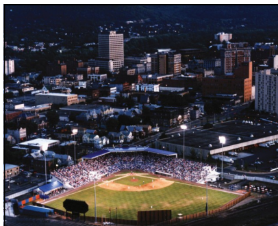
Binghamton Municipal Stadium seen from above in 1992
