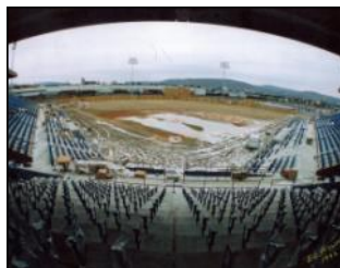
Municipal Stadium under construction in 1992
