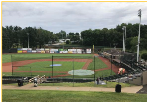
DeVault Memorial Stadium
