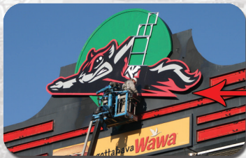
March 7, 2010 Nutzy Scoreboard Construction The Diamond
