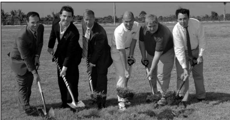
A University-wide ceremony was held to break ground on a new track. Expected completion is Spring 2007.
