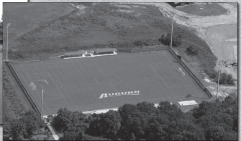
Auburn University Soccer Complex
