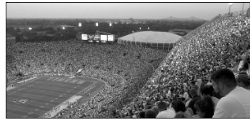
Eastside Expansion of Tiger Stadium
