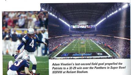
The roof is made of translucent Tefloncoated fiberglass fabric, and takes 10 minutes to open and close. When opening, the roof splits at the 50-yard line and docks in the end zones. The roof can withstand winds as strong as 140 miles per hour when closed and secured. Six of the 16 Texans games have been played with the roof closed, as was Super Bowl XXXVIII.
